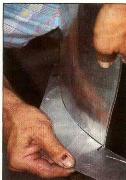
The template is used continuously all along the work piece continually looking for low spots. At the same time the cowlings radius has to be monitored and maintained.
