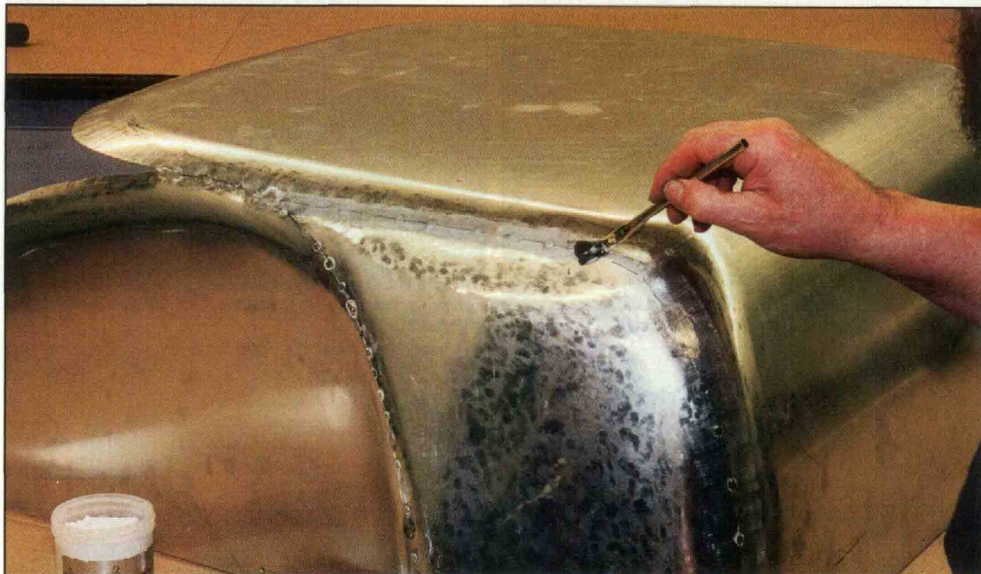
The paste flux for aluminum gas welding is applied with an acid brush.
