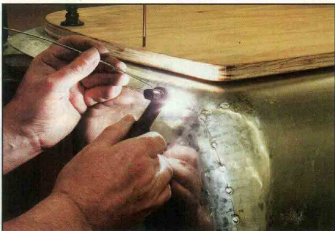
We're using a TIG welder to tack weld the panels together.
